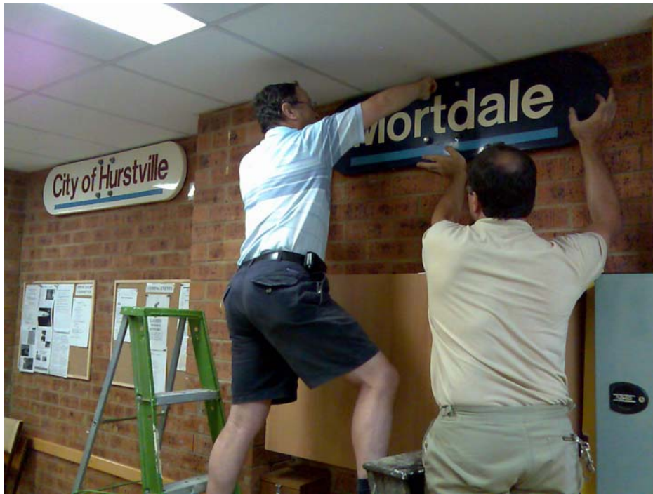
David Bennett and Mic Wade move the Mortdale Station sign in preparation for the installation of an air conditioner in the downstairs meeting room. January 12, 2007.
