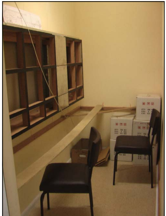
The newly installed CTC panel for Stony Creek. A desk will be installed where the timber has been placed. March 24, 2007. Photo: Glenn Percival
