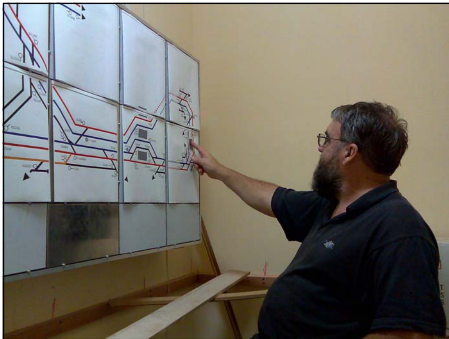
Denis Gilmore explains the future operation of the Stoney Creek CTC panel. Installed in late March, mock-ups of the CTC mimic diagram were soon fixed into position. The plank in front of Denis marks the future location of the CTC operators desk. April 14, 2007. Photo: Glenn Percival
