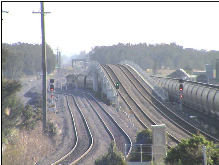
A QR National empty coal train passes under the Sandgate Flyover. Opened late last year, the Flyover allows coal trains access to Kooragang Island from the Up and Down Coal lines (left) without interfering with operations on the Up and Down mainlines which now pass overhead. June 24, 2007. Photo: Chris Winston
