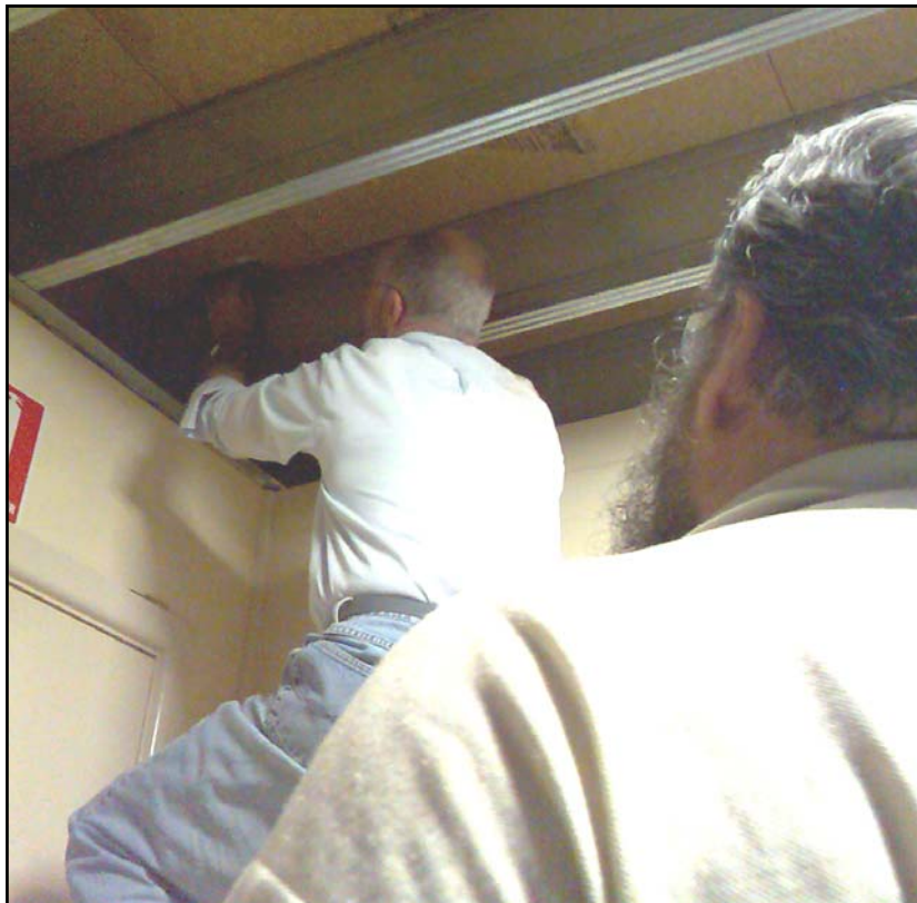
Robert Merrick and Denis Gilmore cut through the first floor to access the HO CTC Room wall space for the running of cables containing 600 pairs of wires. This will "future proof" the CTC Room by providing access to the status of the whole layout, plus spare capacity. June 3, 2007. Photo: Glenn Percival
