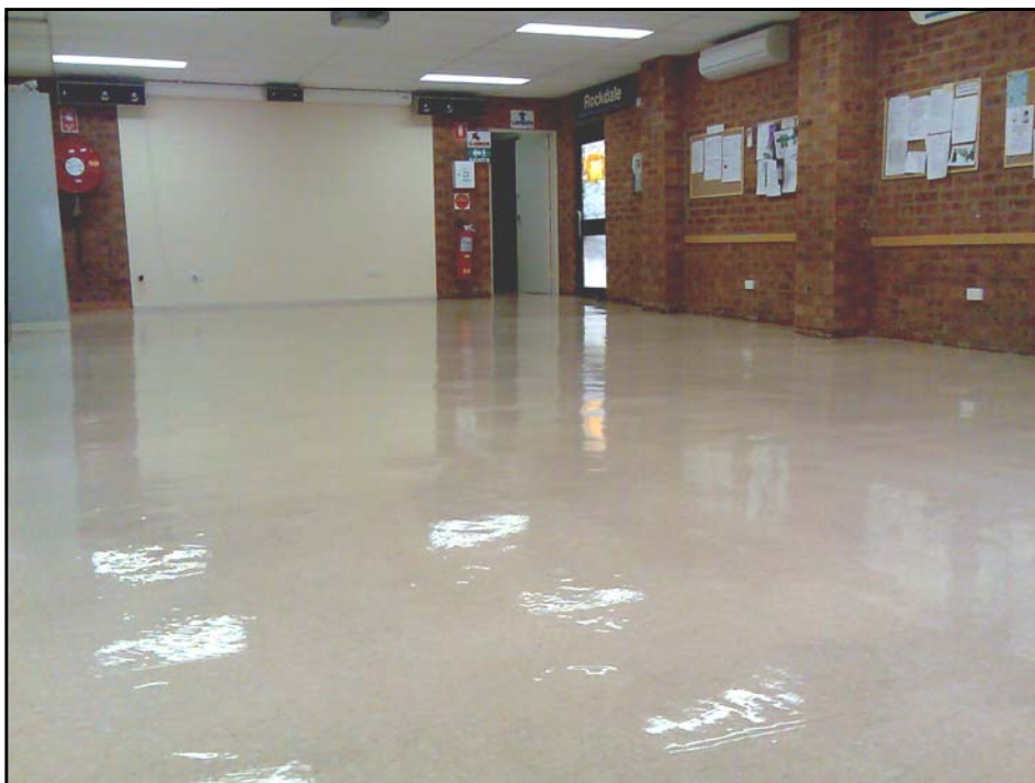
Recent work at the clubrooms has seen the vinyl floor covering cleaned and sealed. The downstairs meeting room shows the rather shiny end result. The big job now is to keep it clean!
