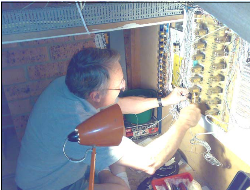
Our dedicated President Barry Wilcockson modifies Stoney Creek Yerrilyong Down Yard's relay panel to implement the departure end shunting neck. January 20, 2007. Photo: Glenn Percival
