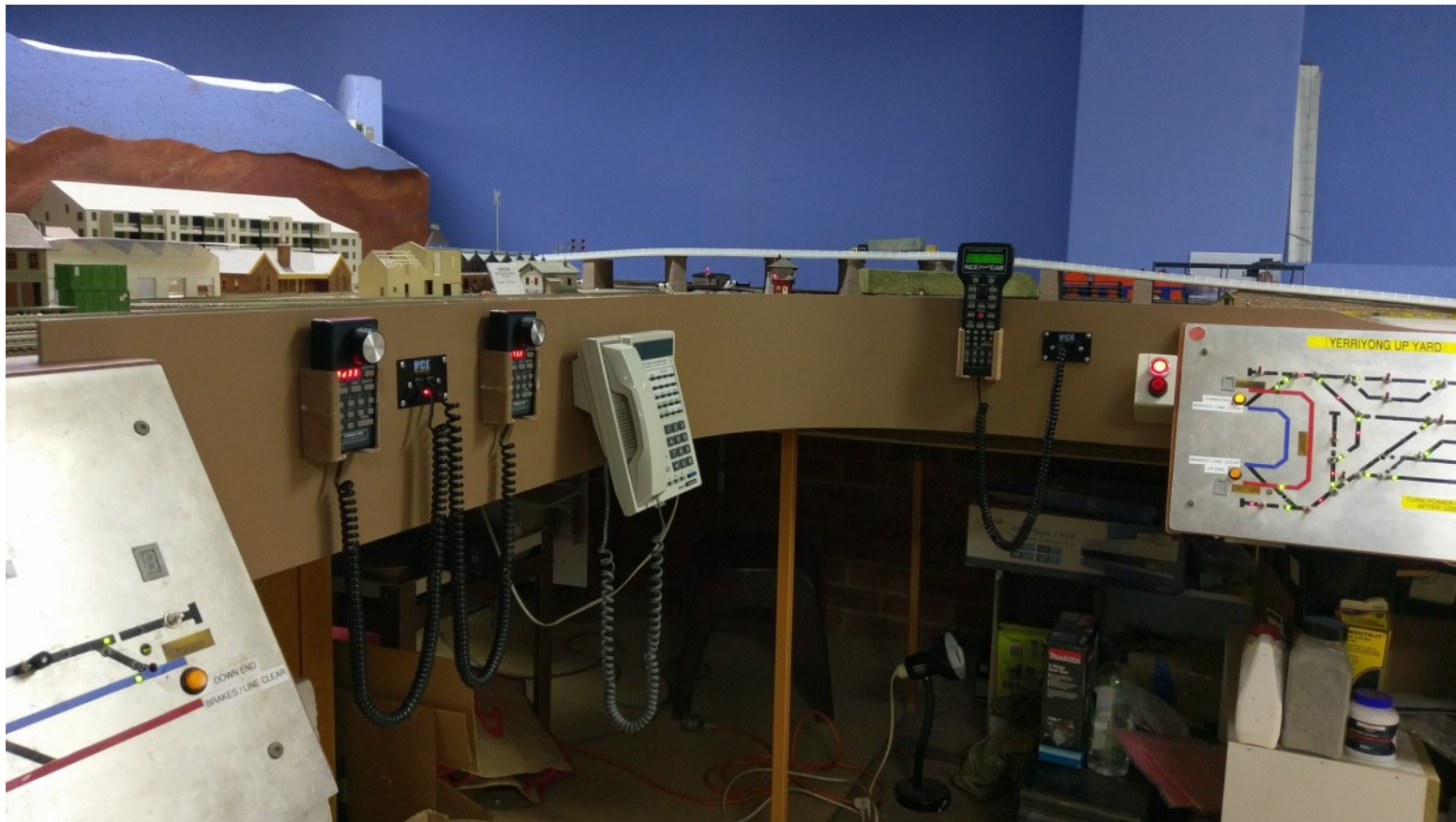
Above: The new facia that has been installed @ Yerriyong. (Thomas Durber)
